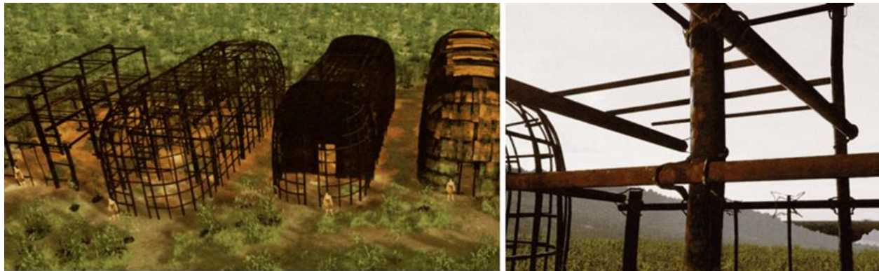
Fig. 4: Layout of sequential phases of longhouse construction from primary structure to finishing envelope (Left). Details within the model showcase the lashing utilized to hold wooden members together (Right).
